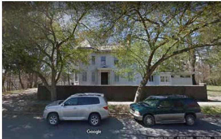
28 Garfield Place. Image from Google Street View.
