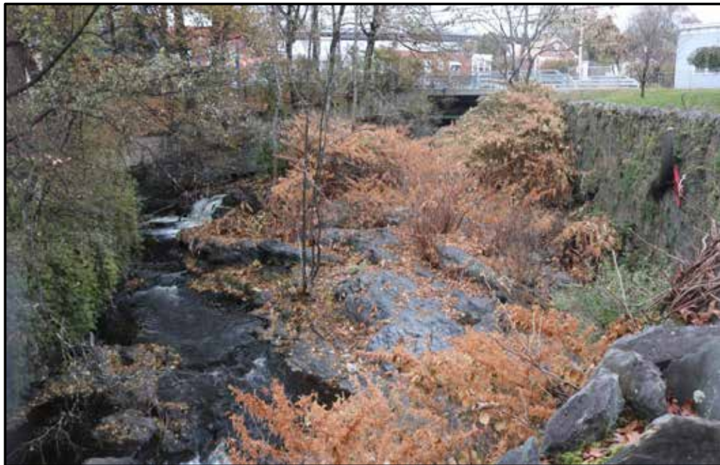
Fall Kill less channelized with natural, rocky streambank. Walls remain and channelize high flows and limit animal access. E. Heffernan © 2018
