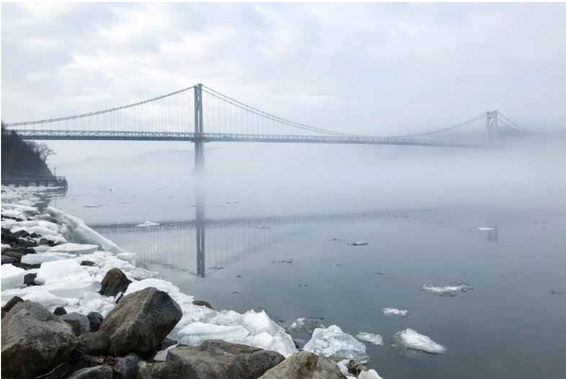
View of the Mid-Hudson Bridge from Waryas Park, Poughkeepsie. Photo credit: Sarah Salem
