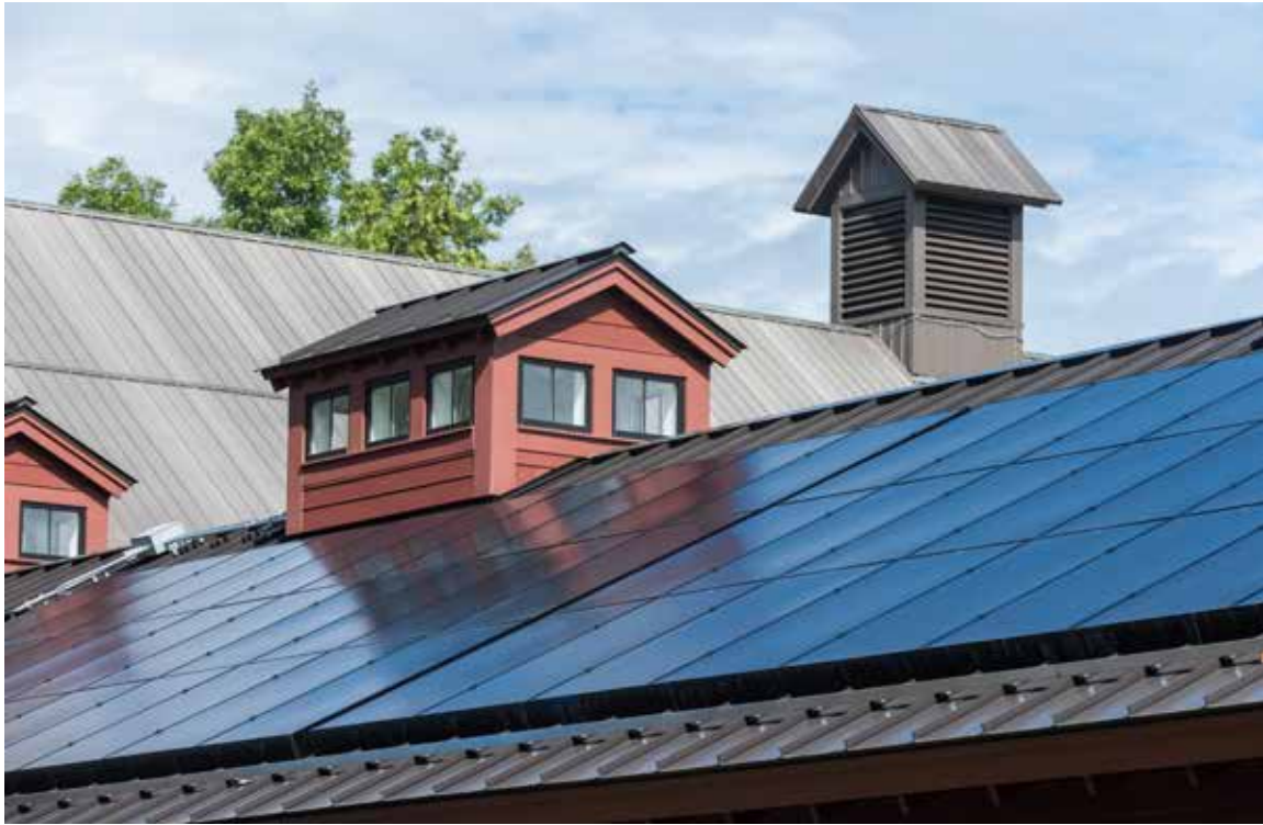
Solar panels at the Environmental Cooperative at the Vassar Barns, Vassar Farm and Ecological Preserve. Photo credit: Karl Rabe for Vassar College
